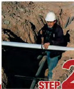
STEP 2 Cut split duct conduit to fit
