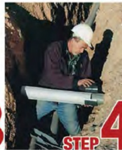
STEP 4 Attach adapters
