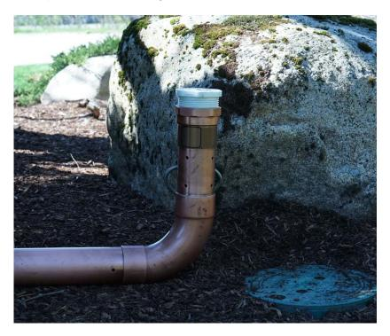
• Chemical rods are often used in conjunction with **soil enhancement materials** that improve grounding effectiveness. These materials can also be used in other grounding systems located in soils with poor conductivity.
