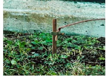
deeper into the earth does substantially reduce resistance. As a general rule, doubling the depth to which the rod is driven into the ground reduces its resistance by up to 40%. However, this has its practical limits.
