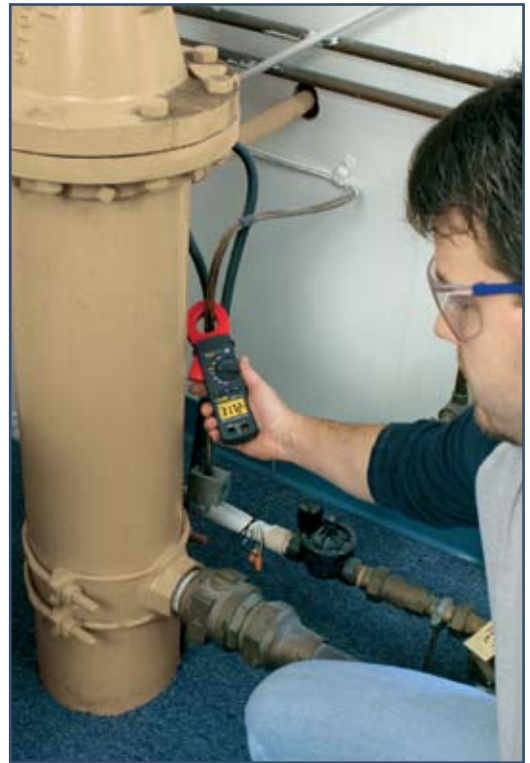
Measuring leakage current on a ground wire with the TRMS Leakage Current Meter Model 565
