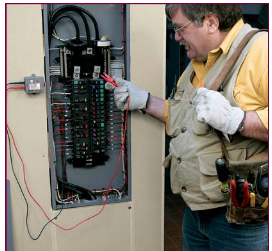
Model L260 setting up to log voltage in a distribution panel.
