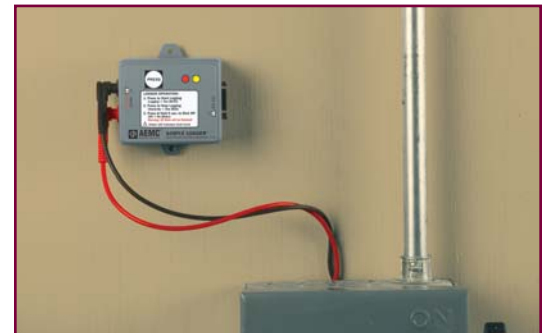
Model L215 monitoring a control panel looking for dropouts and spikes in the line voltage
