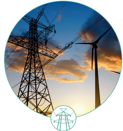
ELECTRICAL POWER TRANSMISSION AND DISTRIBUTION
