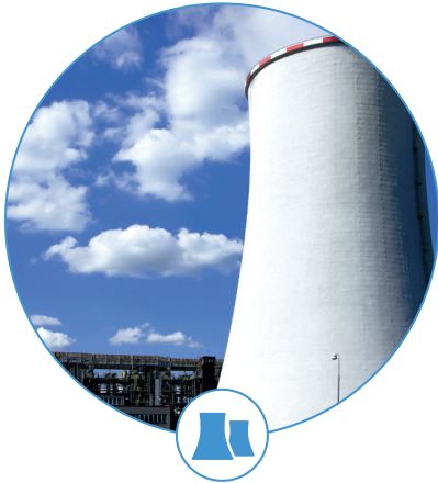
ELECTRICAL POWER GENERATION
